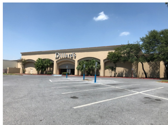
Acquisitions: (Top) A 187,392-square-foot warehouse in Laredo, Texas. (Bottom) A big-box anchor building at a mall in Harlingen, Texas
